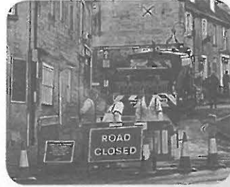
5 Repairs to streets and freeways. (4, 4)
